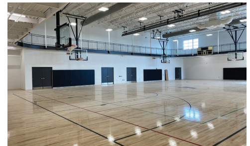
Actual photos of construction in progress: Aquatic Center featuring an 8-lane 25-yard competition pool and a warm water family/class pool and Gymnasium with Indoor Track, Basketball, Volleyball, and Pickleball.
